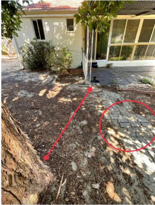
Lifting pavers & distance from tree to Concrete.
