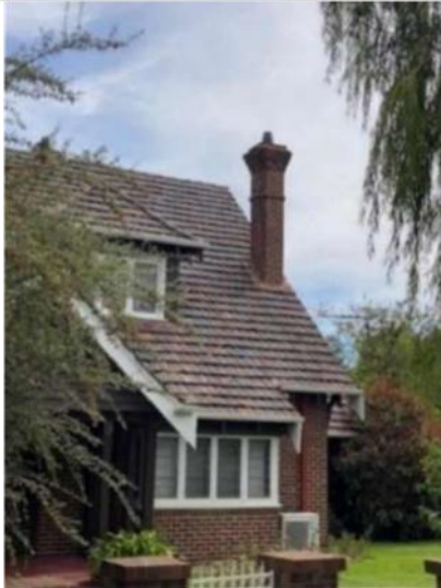
Onslow Street elevation (2024)
