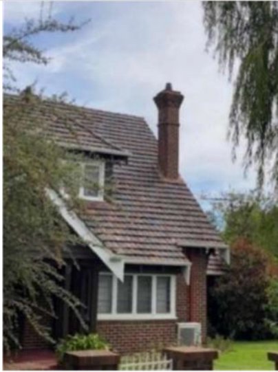
Onslow Street elevation (2024)
