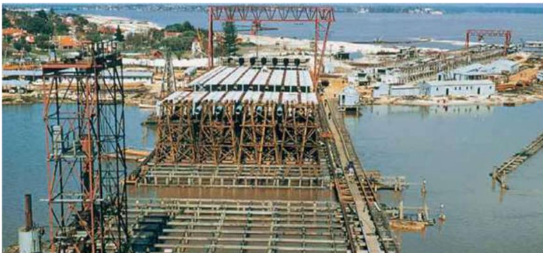
Figure 28 Narrows Bridge under construction, c1958. Courtesy: Picture South Perth Photographic Collection
