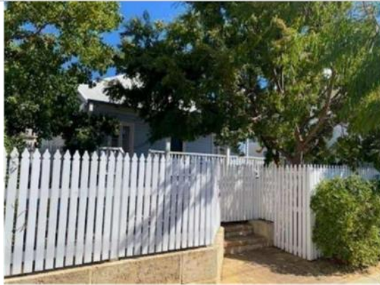
No. 29, Strata Lot 1 (Front) Hovia Terrace (2024)
