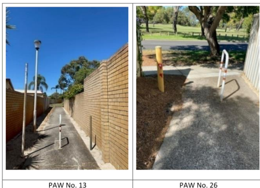
Figure 12 Images of PAWs showing insufficient clearance around bollard structures for universal access.
