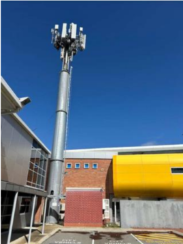
Image 3: Ground level photo of the existing telecommunications facility (facing west).
