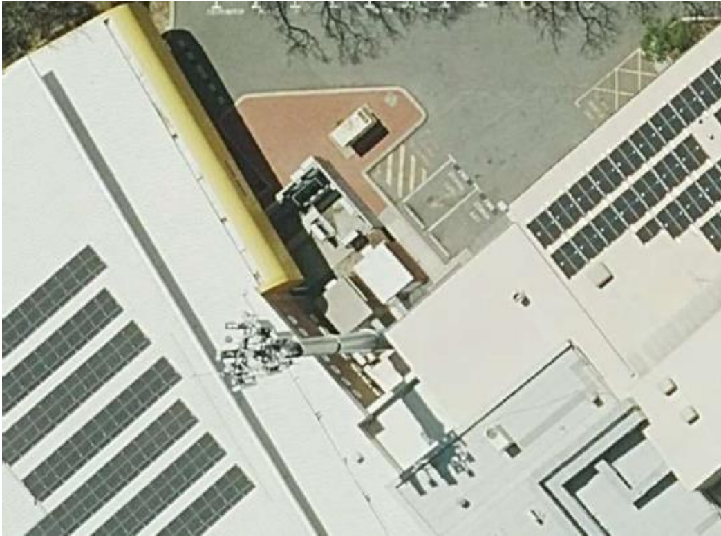
Image 1: Aerial photo of the existing telecommunications facility.
