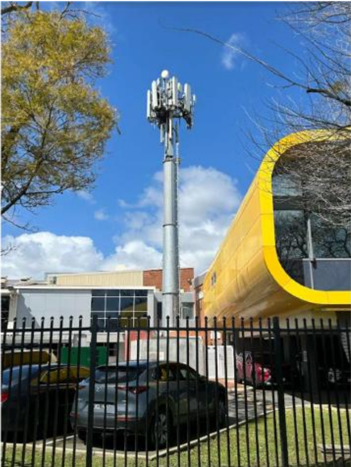
Image 2: Ground level photo of the existing telecommunications facility (facing south).
