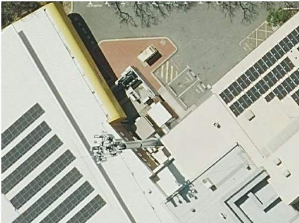
Image 1: Aerial photo of the existing telecommunications facility.
