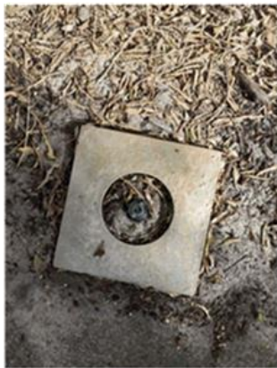
Reticulation Sprinkler Heads (Distributed beside length of footpath)
