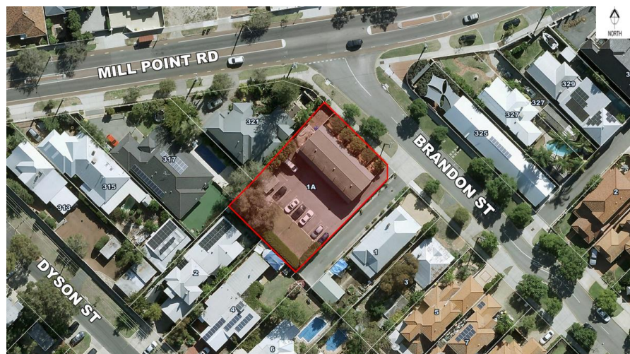
Figure 1: Aerial image of site
