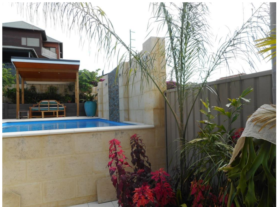
Figure 5: Limestone dividing fence abutting pool area, as viewed from 63 Gwentyfred Road.
