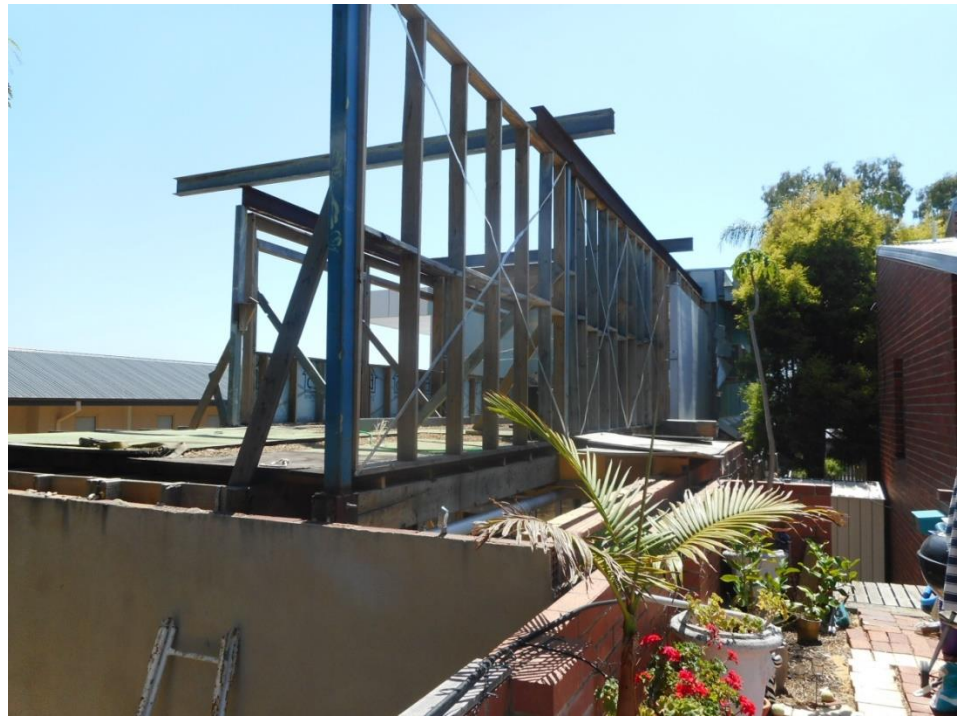
Figure 4: View of south-east elevation of No. 22A Banksia Terrace, from the perspective of the rear of 24 Banksia Terrace. This image shows the rear portion of the building (partially) constructed with a south-eastern setback of 1.3m. It is proposed to be altered to 2m.
