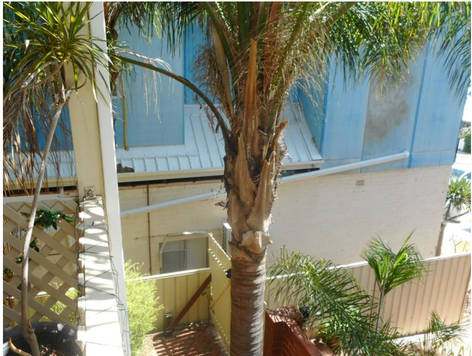
Figure 6: An example of some external piping on south-eastern elevation of subject site, as viewed from the balcony at 24 Banksia Terrace.
