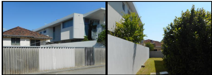
Figure 3: Images of Side Boundary Fence between subject site and No. 27 Waverley Street and Right-of-Way fence
