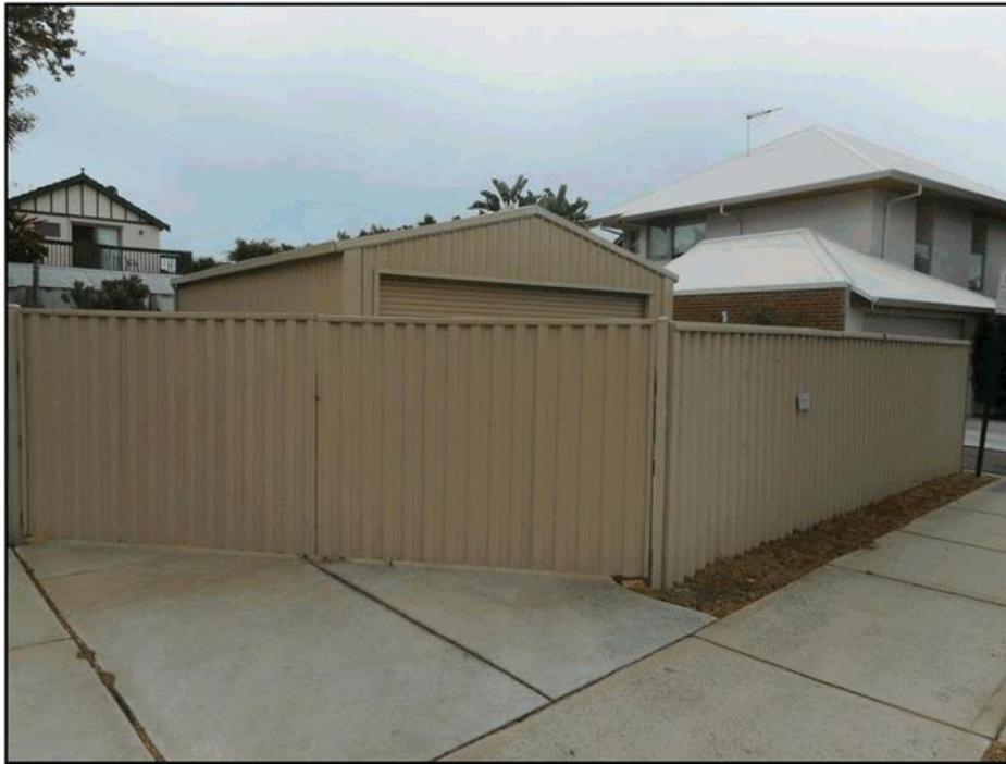
Site photo of existing outbuildings as viewed from Sandgate Street
