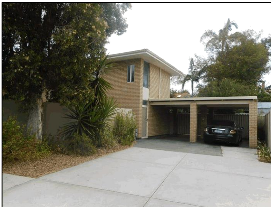
Site photo of Multiple Dwelling as viewed from Sandgate Street
