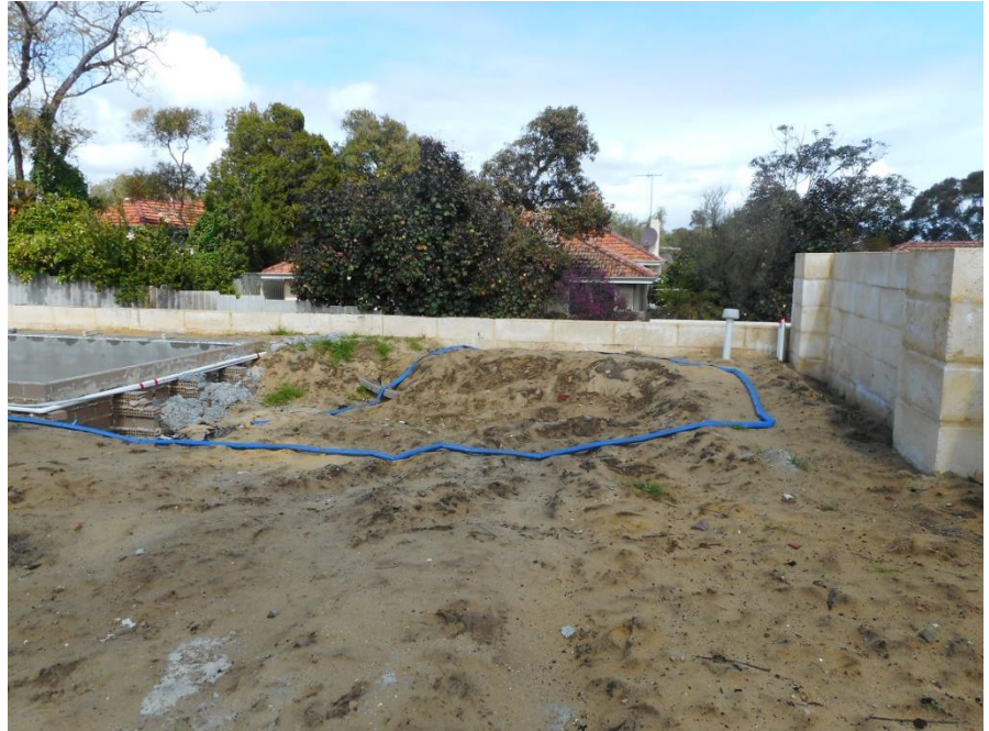
Figure 3: Site works at the rear of the subject site.
