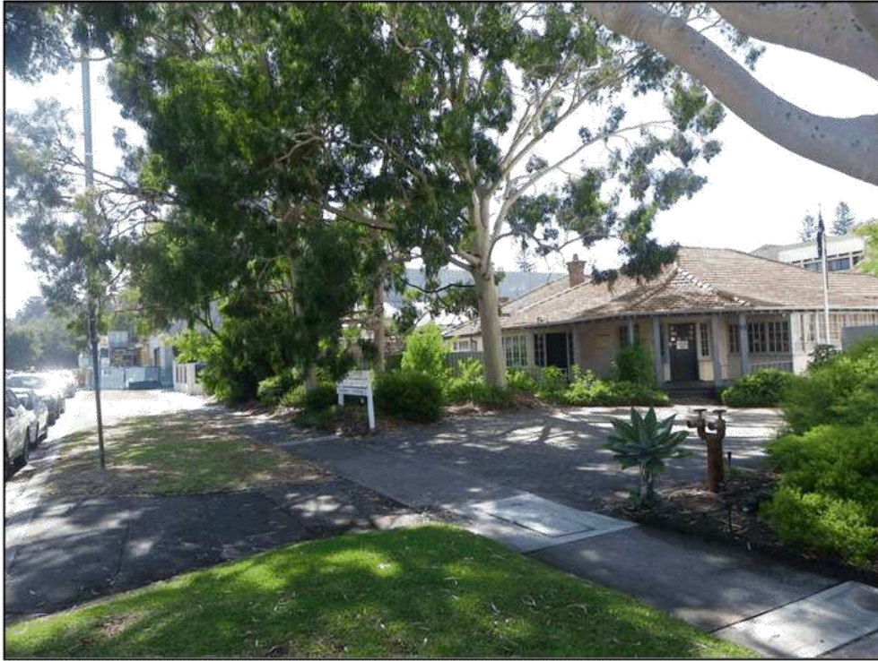
26 Charles Street - View from Charles Street, facing south east (February 2016)
