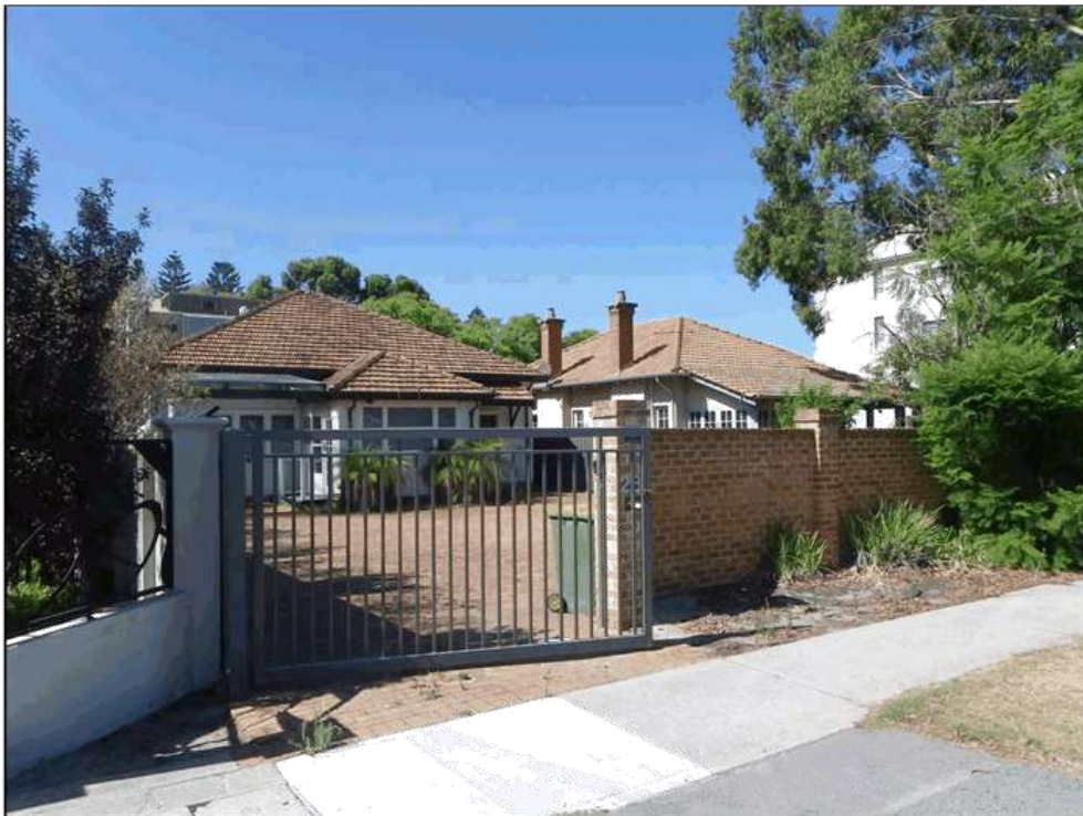
28A (Left) & 26 (Right) Charles Street - View from Charles Street, facing south (February 2016)
