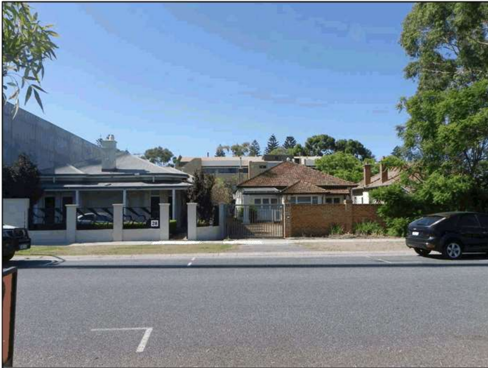
28 (Left) & 28A (Right) Charles Street - View from Charles Street, facing south east (February 2016)
