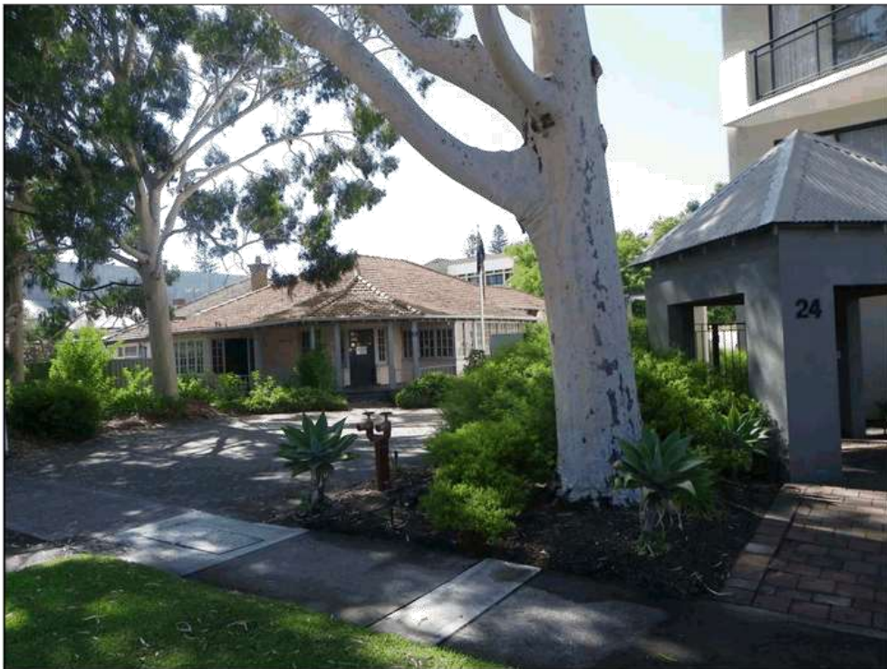
26 (Left) & 24 (Right) Charles Street - View from Charles Street, facing south east (February 2016)
