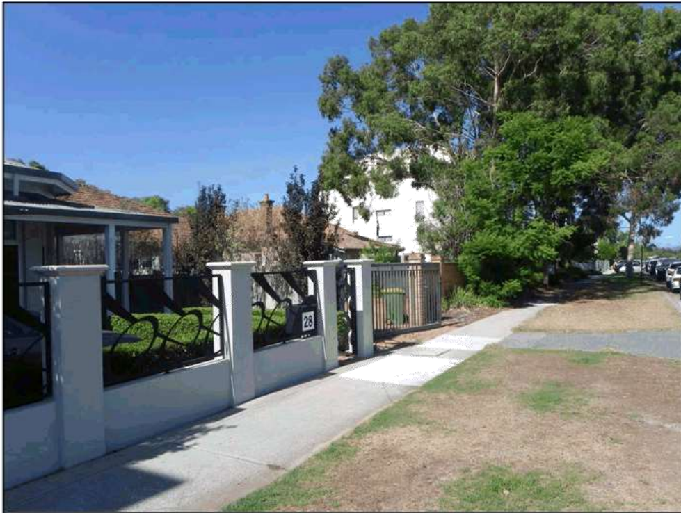
28 (Left) & 28A (Right) Charles Street - View from Charles Street, facing south west (February 2016)
