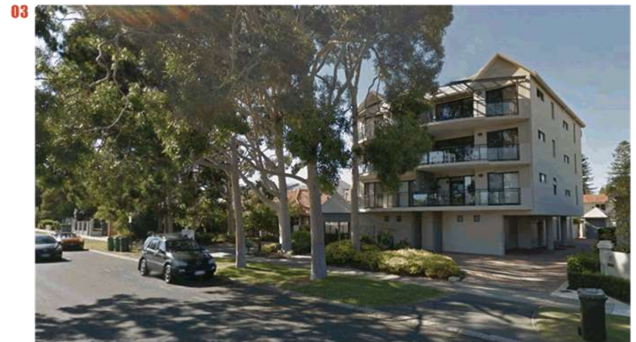
Street Scape view from adjacent property
