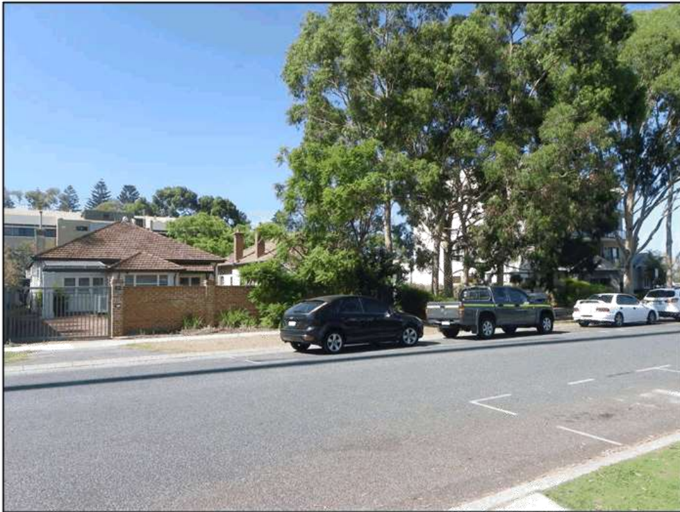
28A (Left), 26 (Centre) & 24 (Right) Charles Street - View from Charles Street, facing south (February 2016)
