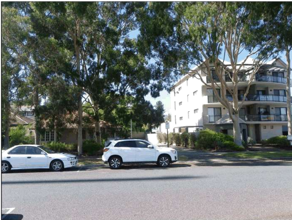
26 (Left) & 24 (Right) Charles Street - View from Charles Street, facing south east (February 2016)
