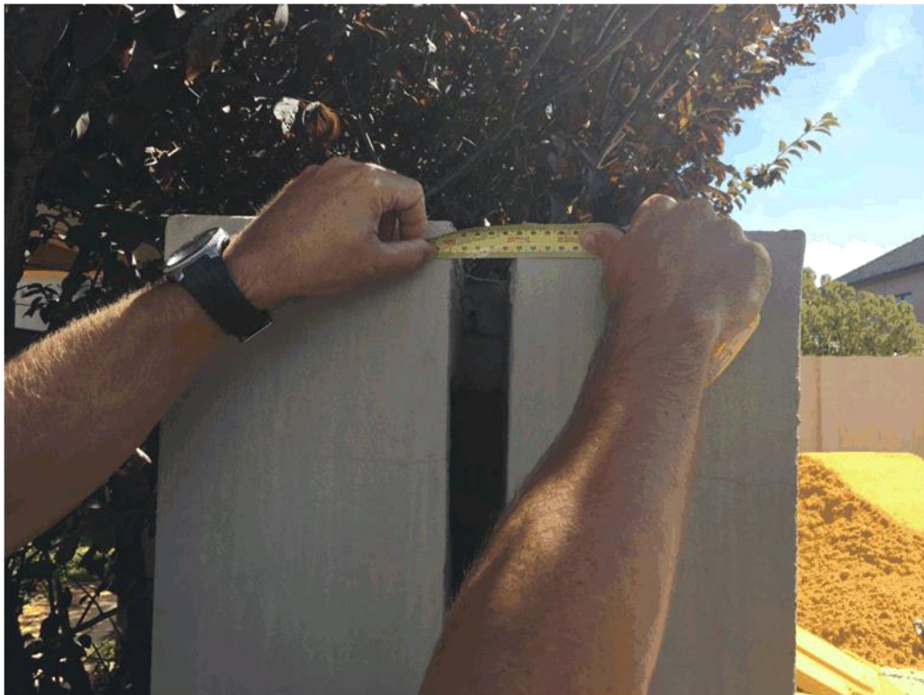
PHOTOGRAPH 2 – APPROXIMATELY 50MM OFFSET AT TOP OF WALL
