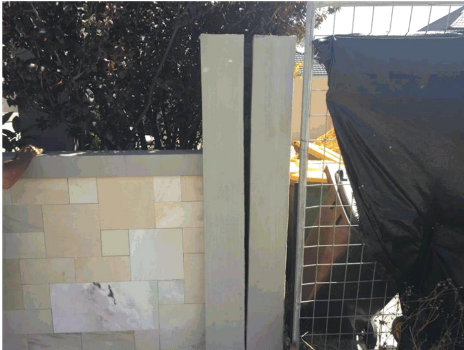
PHOTOGRAPH 1 – OVERVIEW OF ROTATED WALL (RIGHT) RELATIVE TO PLUMB WALL (LEFT)
