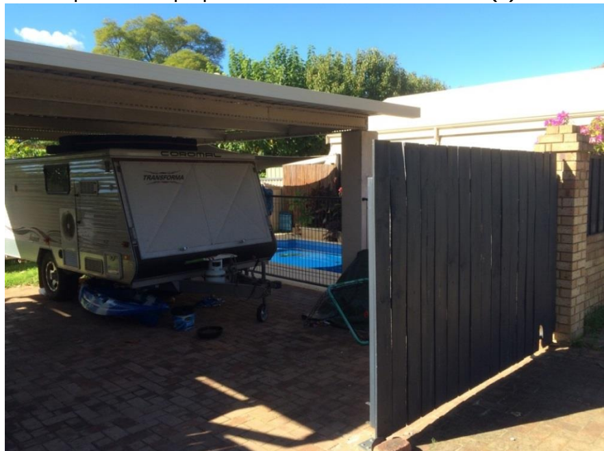
Photo I - The image shows the existing carport structure on the subject site.
