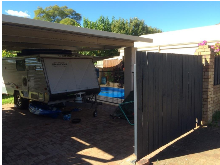
Photo 1 - The image shows the existing carport structure on the subject site.
