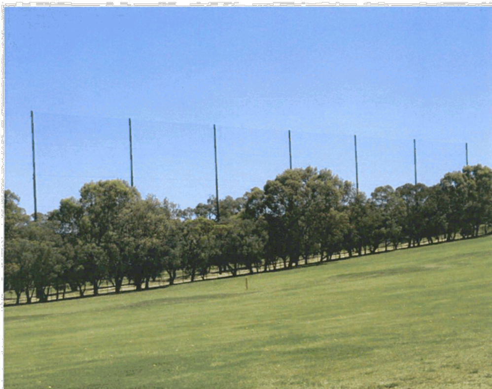
Wembley Golf Course - Perth. At up to 36m tall this is one of the highest engineered fences in Australia and has set new design parameters for both poles and footings in this country.
