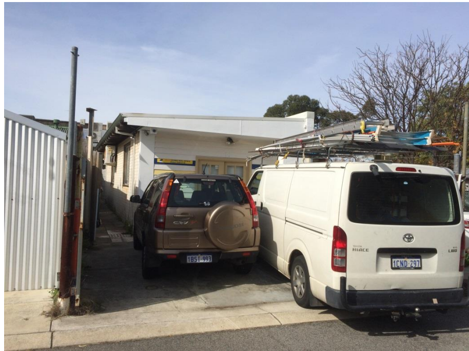
Photo 1 - Existing office at rear of 8 Moresby Street
