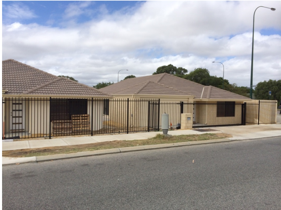
Site Photo I – Completed Single House being proposed as Display Home
