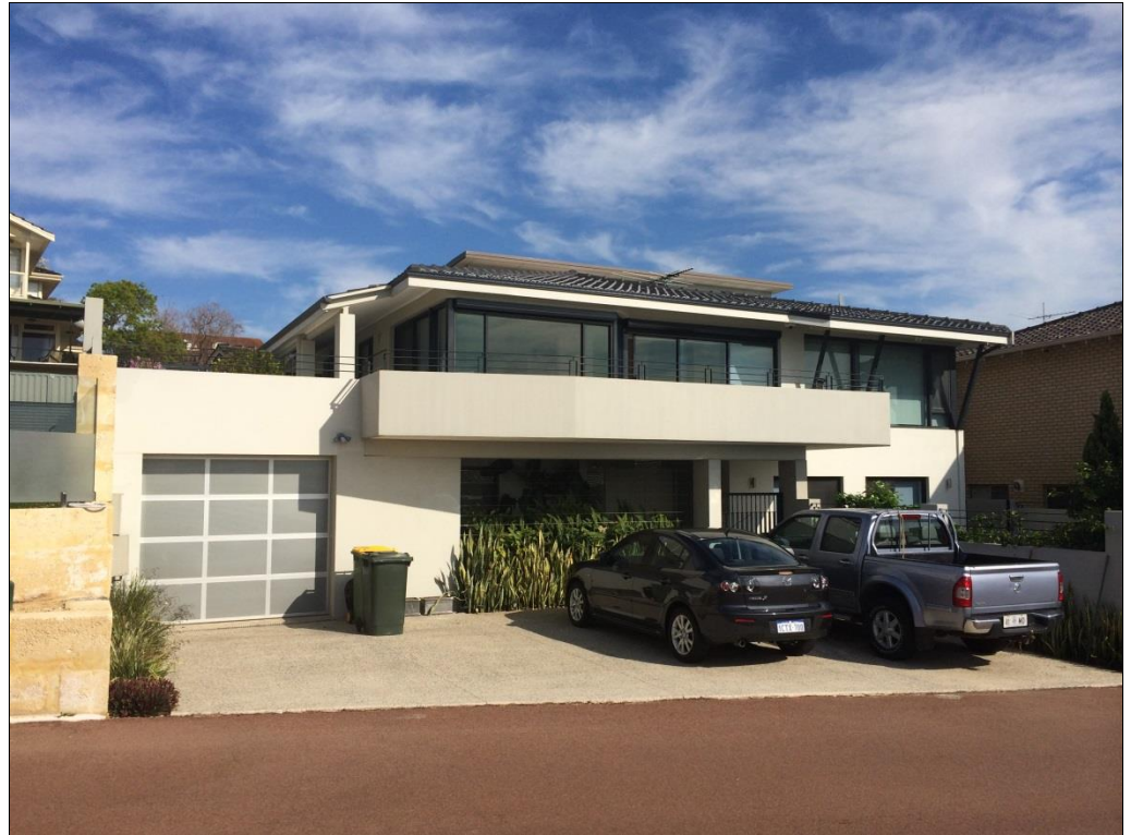
Site Photo 1 – Existing River Way elevation.
