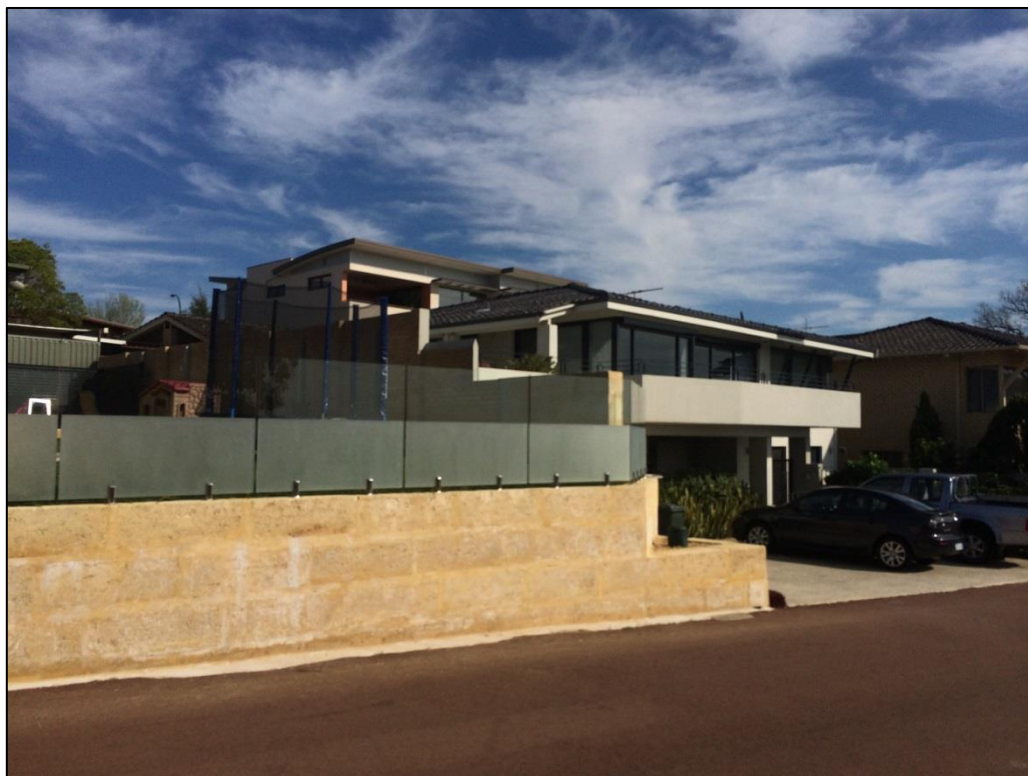
Site Photo 6 – Existing limestone wall and fencing structure adjacent to the subject site.
