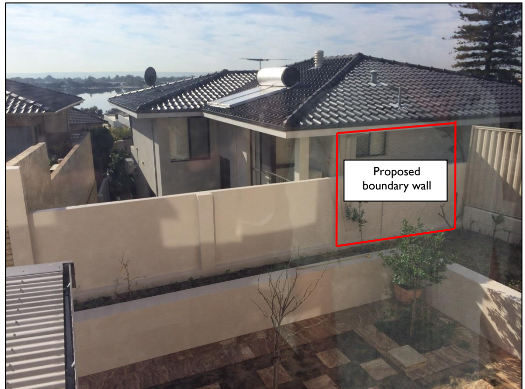
Site Photo 2 – View from the first floor at 29 Howard Parade (dining).
