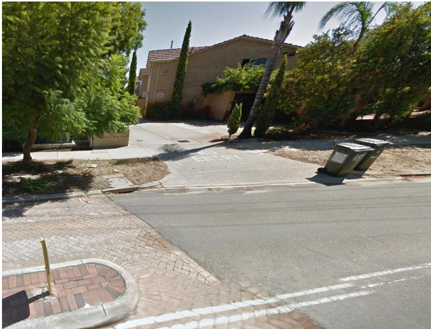
Units to the North at 87 Ley Street
