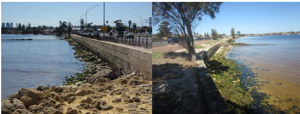
Plate 10: Skinny Foreshore (a) middle facing north (b) middle facing south
