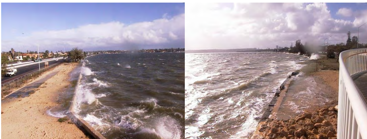
Plate 1: Photos After the Peak of the May 2003 Storm. Thelma Street Footbridge looking South and North.
