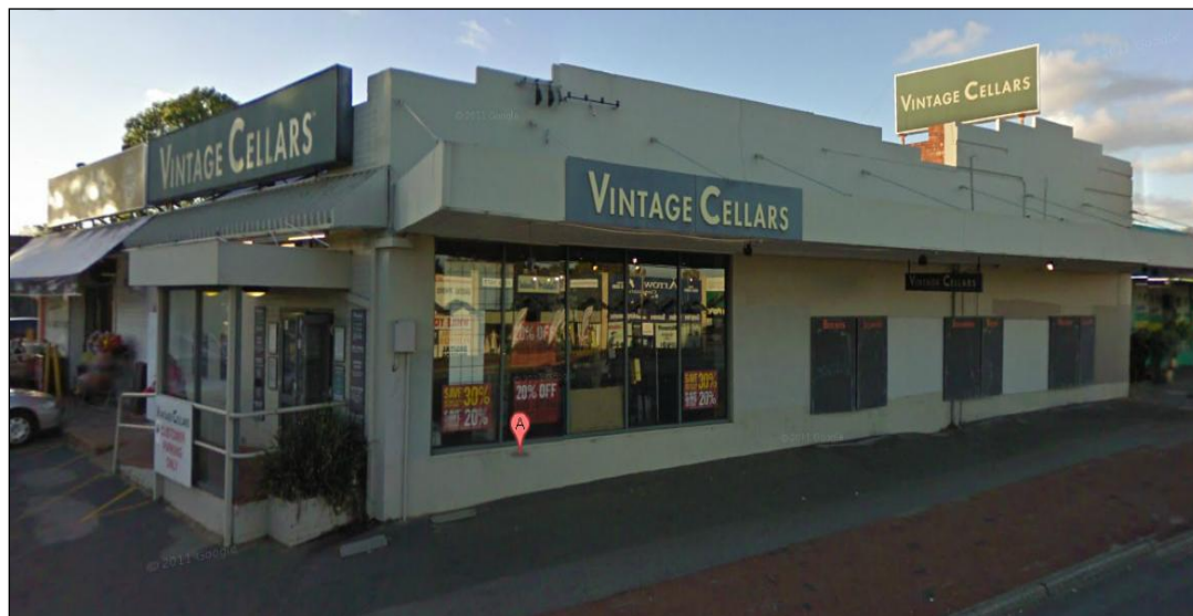
Figure 1 - Site photos 2010 (The previous liquor shop)
