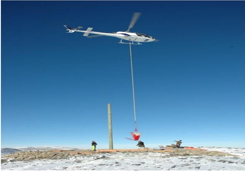
Concrete lifted by copter to multilateration site, Omarama
