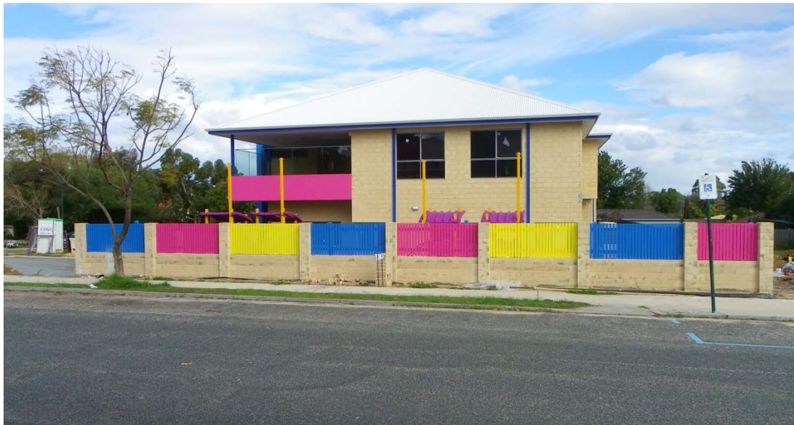
The site as viewed from Alston Avenue
