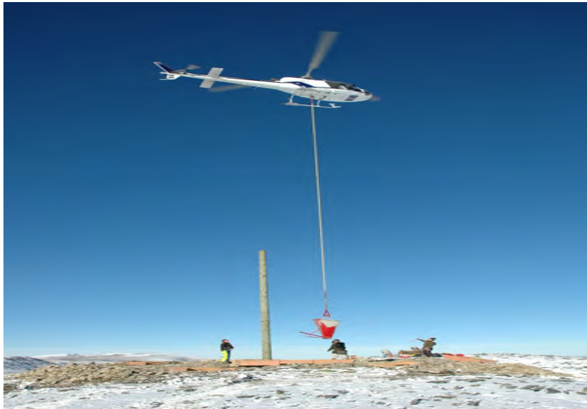
Concrete lifted by helicopter to multilateration site Wether Range, Omarama
