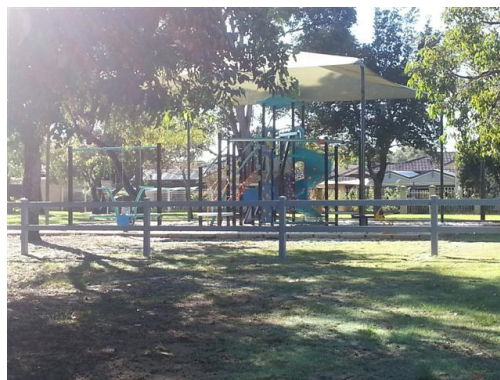
Photograph 2: New Playground & Fence
