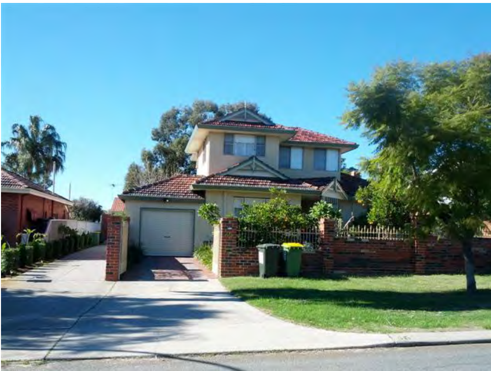
Two Storey Dwelling – 46A Edgecumbe Street.
