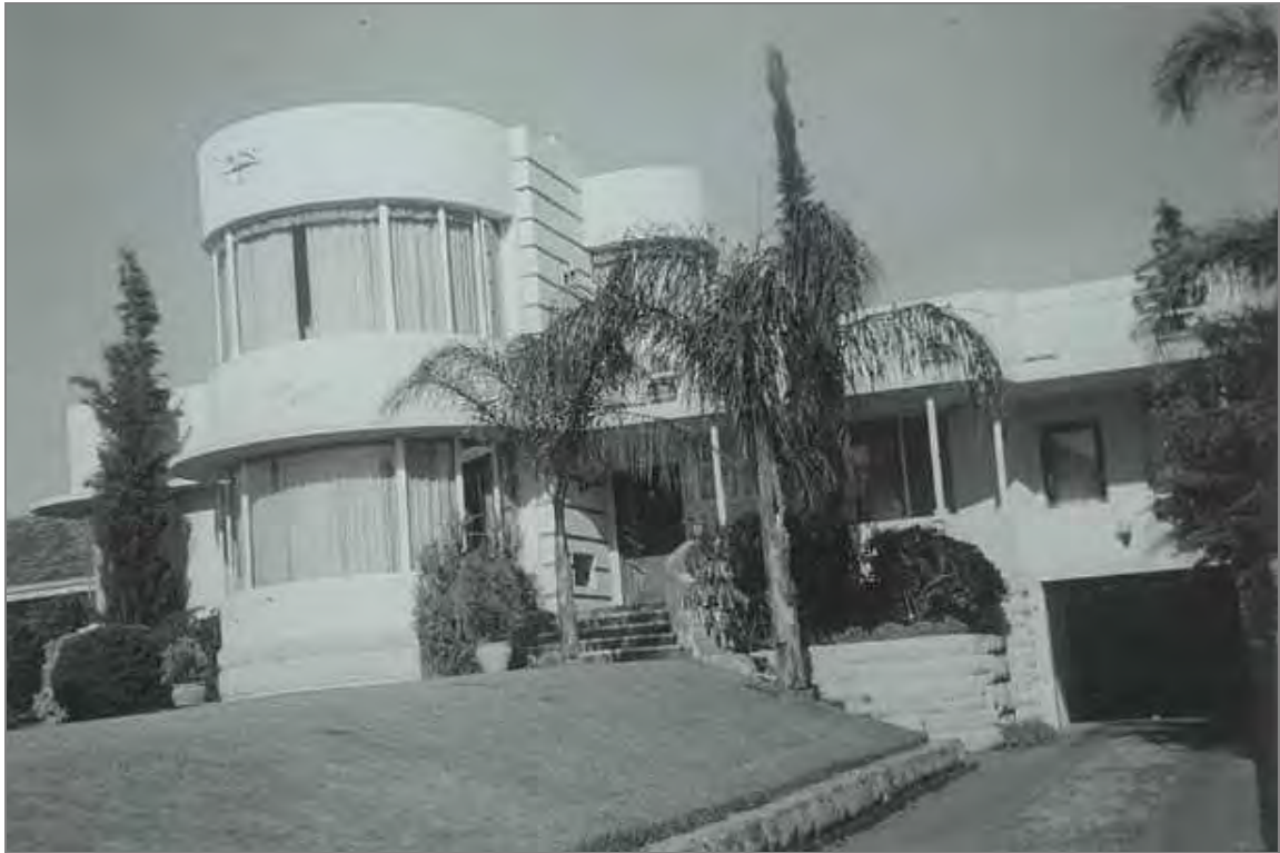
View of the classic front garden and Residence: 426 Canning Highway - 'Blue Waters' c1960. (Courtesy of Mr David Cavanagh, 2006 owner.)
