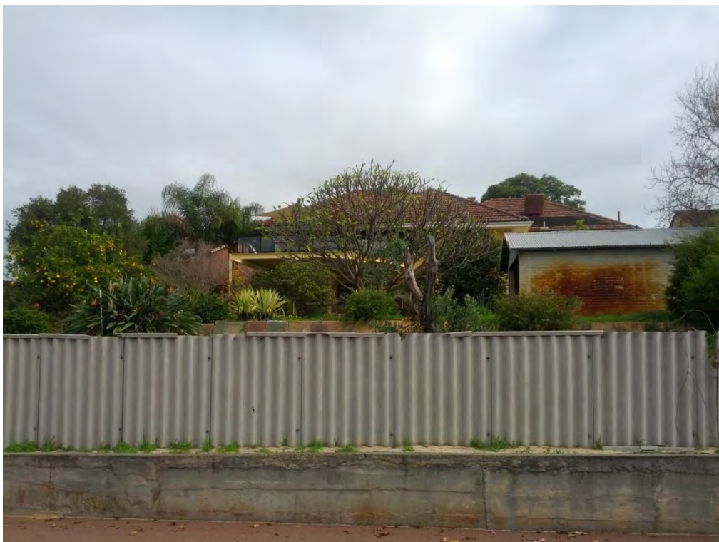
Rear of dwelling at 54 Sulman Avenue, Salter Point
