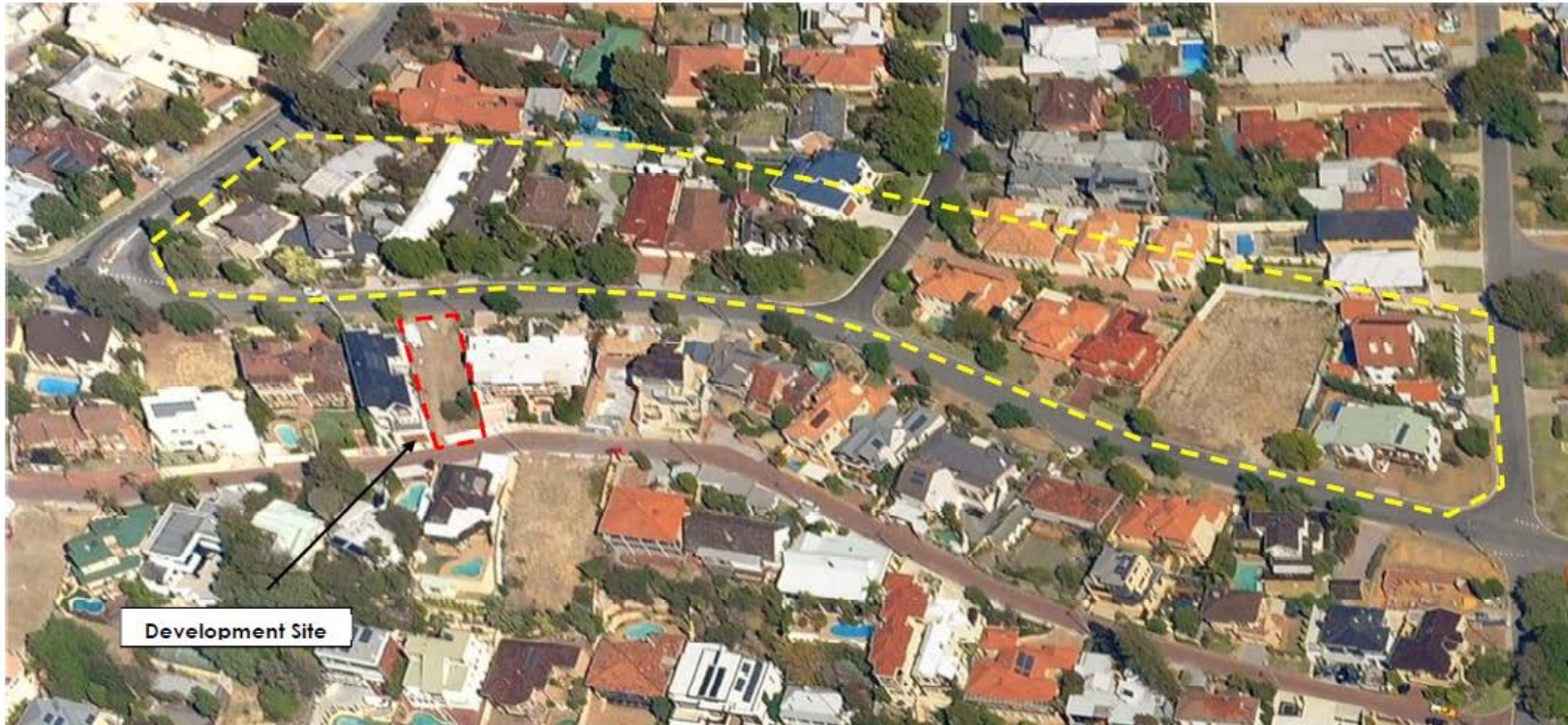
Roof forms opposite the site along Sulman Avenue - West Elevation
