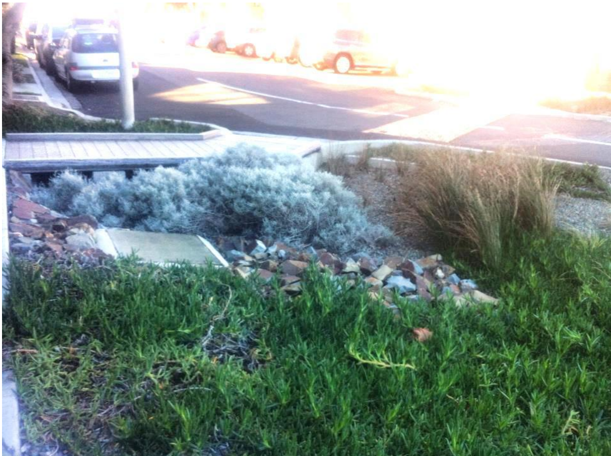
Rain Gardens to combat storm flooding events - Dow Street Water Sensitive Urban Design project which also incorporates landscape design.
