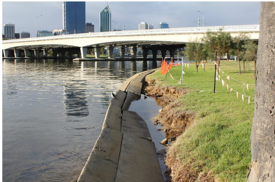
Figure 4 - Deteriorated condition of the river wall
