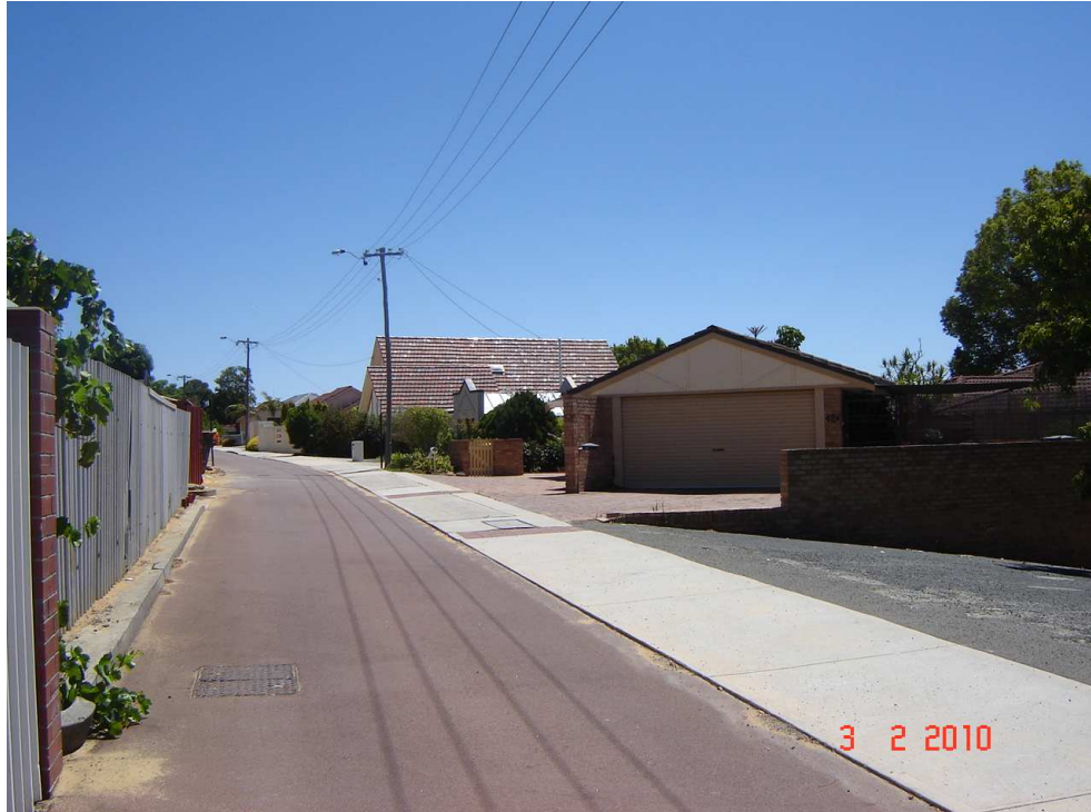
River Way (north)
