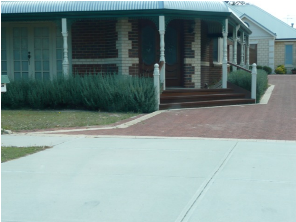
Figure 2 - View from Anthony Street showing steps and railing
