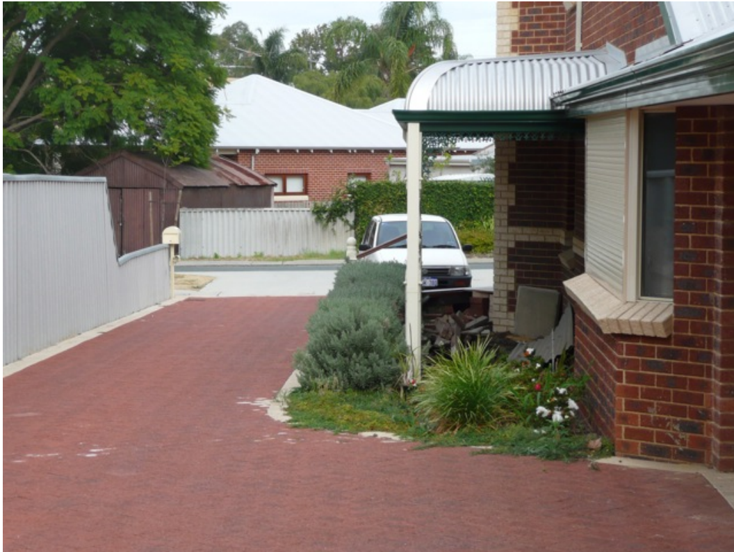
Figure 3 - View from 10A Anthony showing railing protruding over the easement
