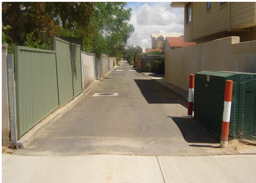
Portion of ROW 109 (looking south)
