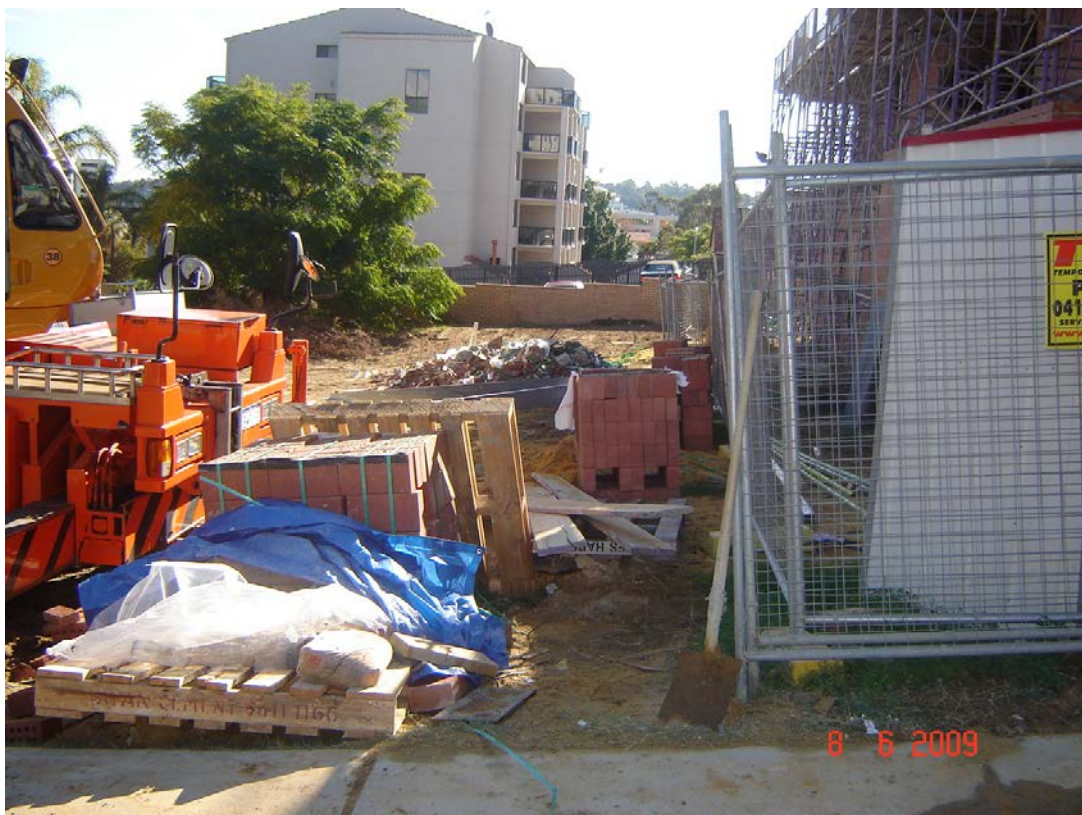
Lot 2 (No. 3) Parker Street, South Perth- front (North West) of site
