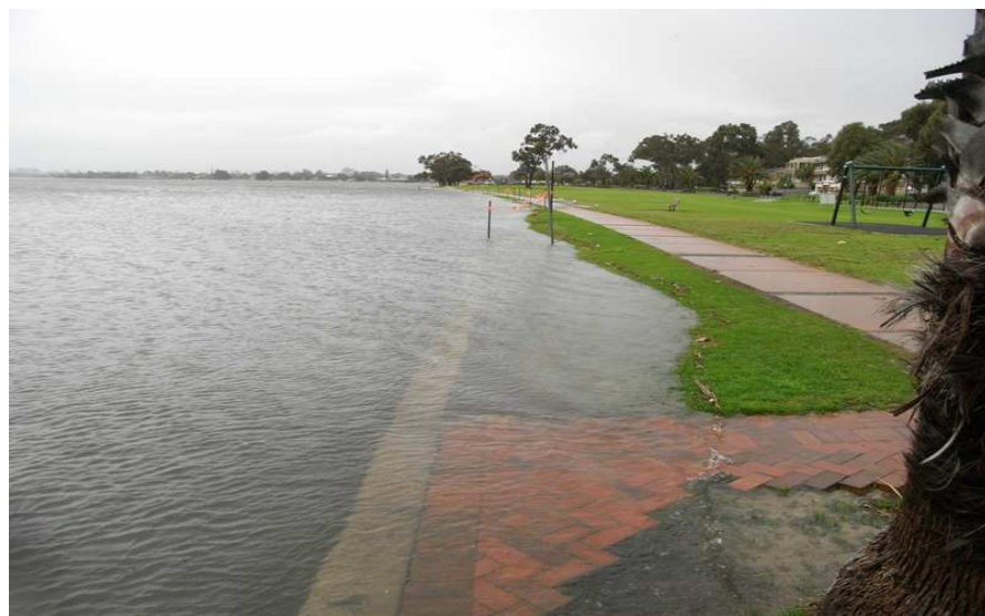
Figure 4. Overtopping of river wall east of Mends Street - July 2008
