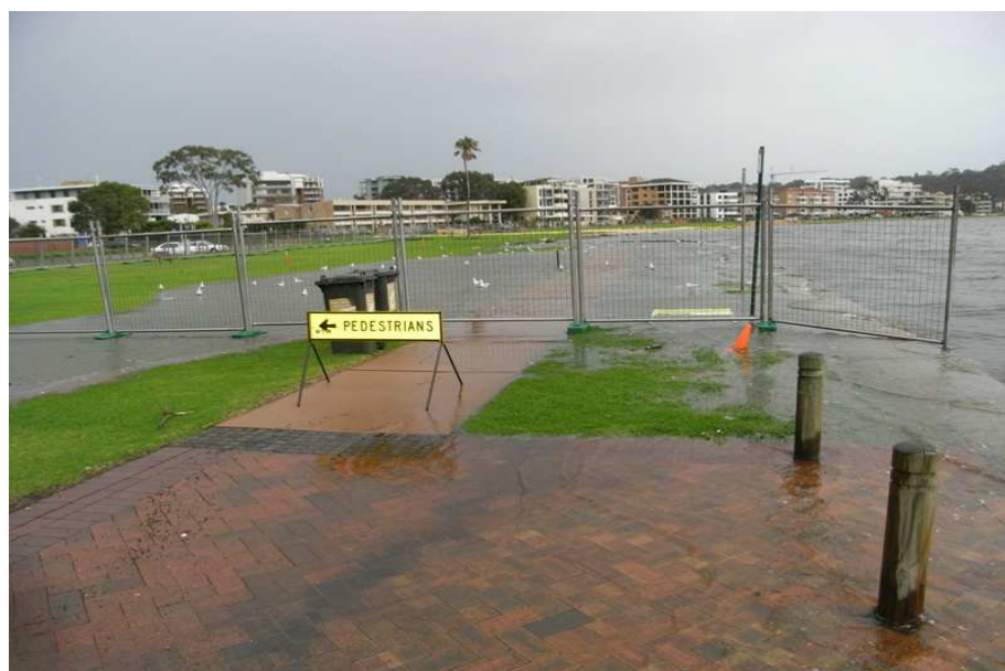
Figure 5. Overtopping of river wall west of Mends Street - July 2008
