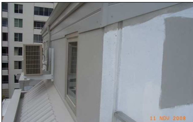
Figure 15: Level 5 window to “Void” - Closed.
