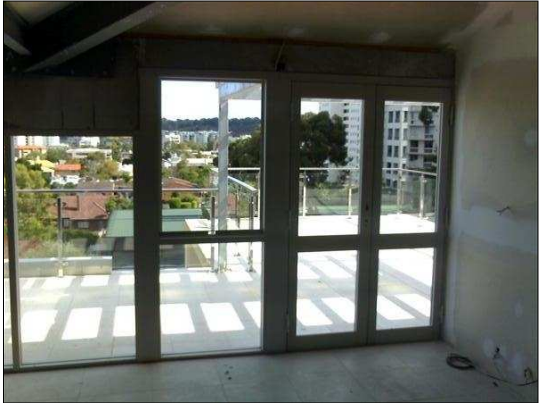
Figure 12: Enclosure of Level 5 “Balcony”.
