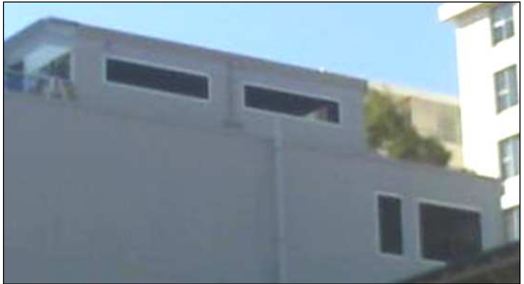
Figure 4: As-constructed Levels 4 and 5 “Balconies” - Site photograph.
