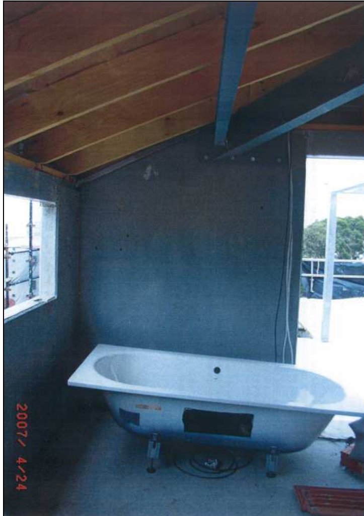
Figure 11: Enclosure of Level 5 “Balcony”.
