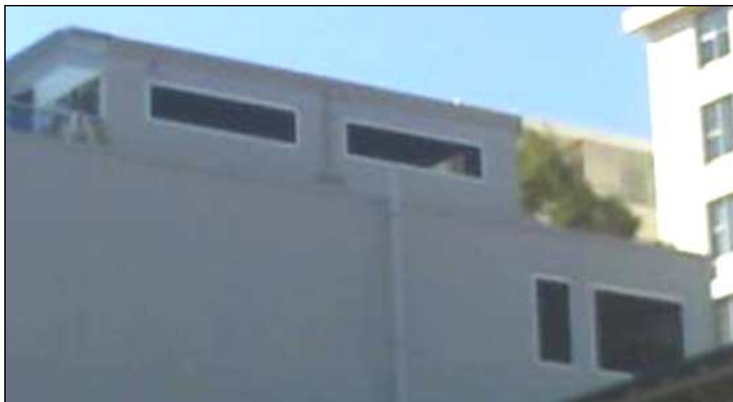
Figure 4: As-constructed Levels 4 and 5 “Balconies” - Site photograph.
