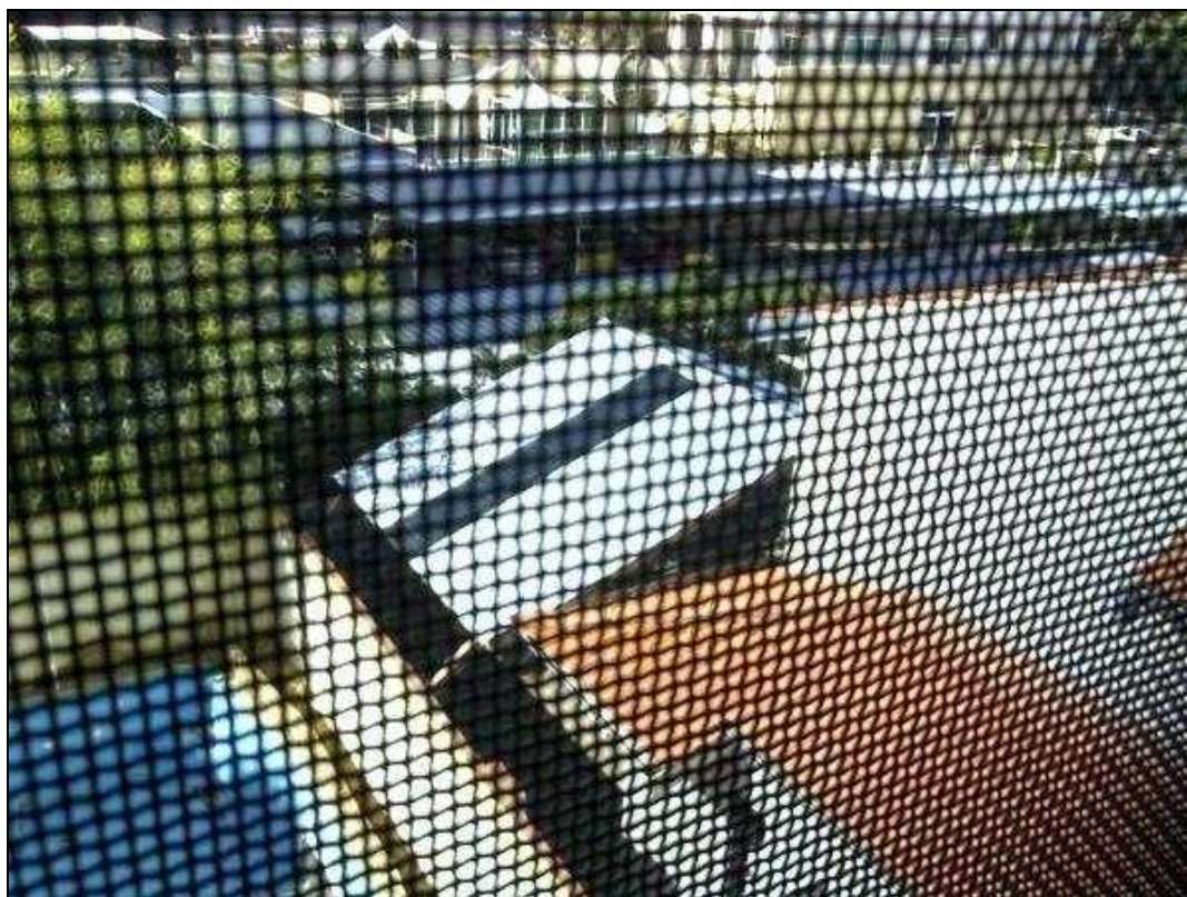
Figure 6: Enclosure of “Balcony” with security mesh.
