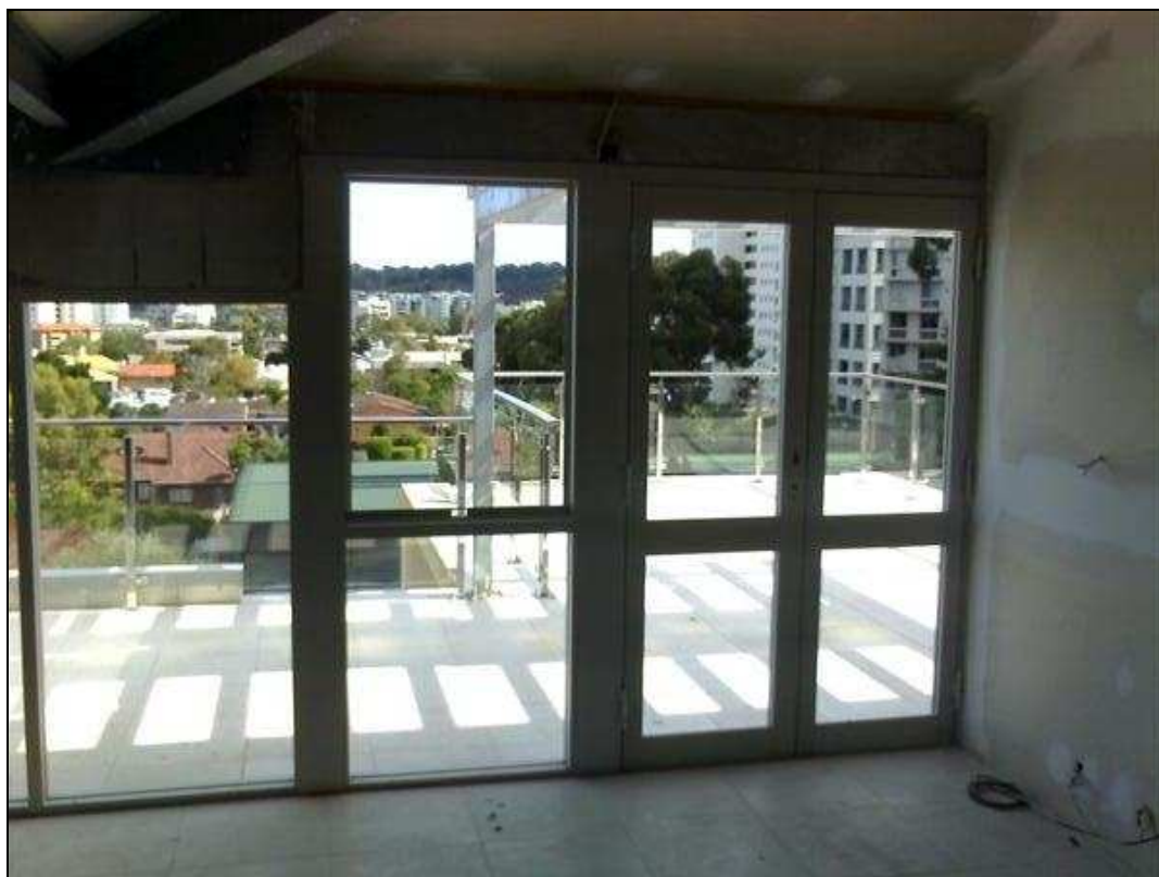
Figure 12: Enclosure of Level 5 “Balcony”.
