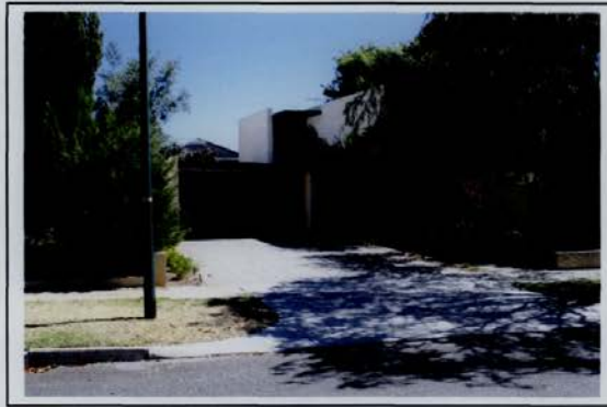
FIGURE 5 – View of Garage Skillion of 17 York Street from York Street
