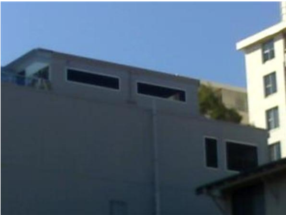
Lot 10 (No. 6) Parker Street, South Perth - Upper 'Balconies'
