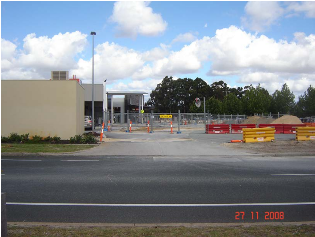
Waterford Plaza, Karawara - north end
