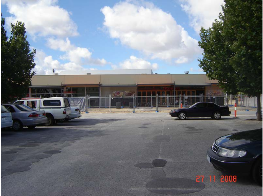
Waterford Plaza, Karawara - south end
