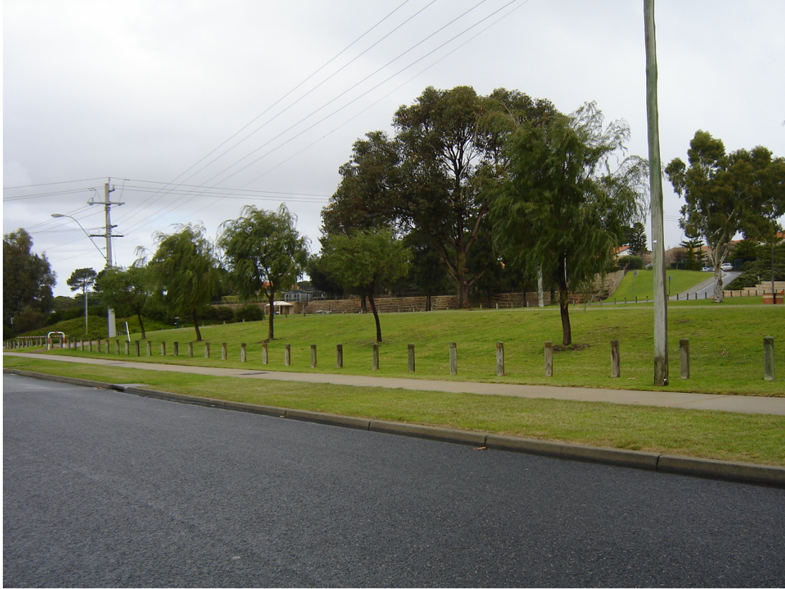
Penrhos College, showing retaining along school side of oval
