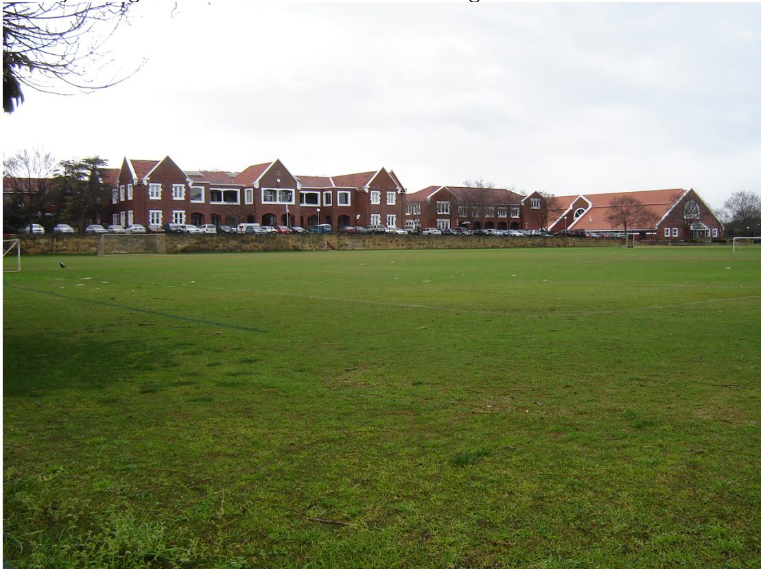
Wesley College, showing retaining wall at school side of oval
