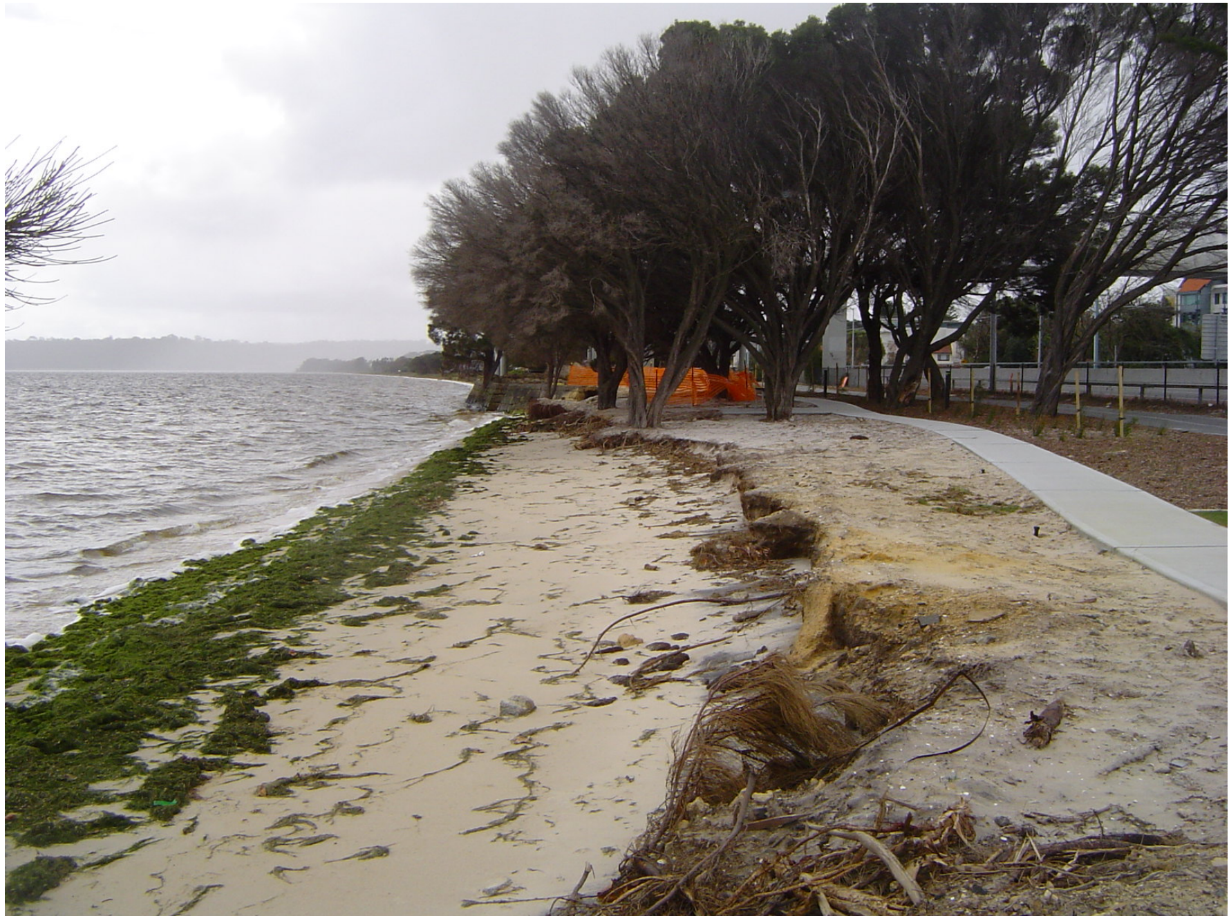
View of Como Beach foreshore looking north to the Comer Street Pedestrian Overpass
