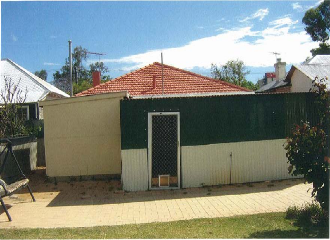
Photo 3- Existing enclosed patio and outbuilding
