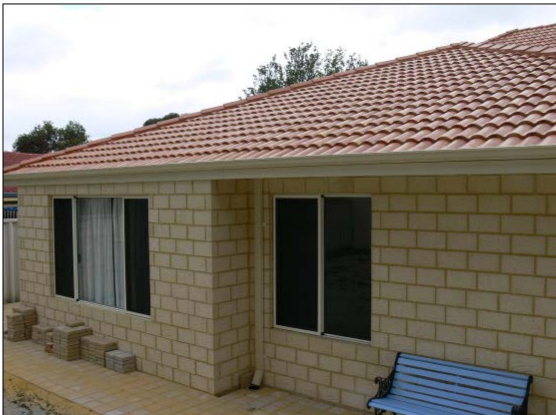
View of rear wall of house which will face the shed.
