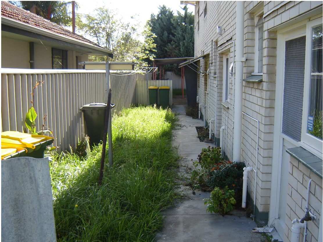
Side of building from other end
