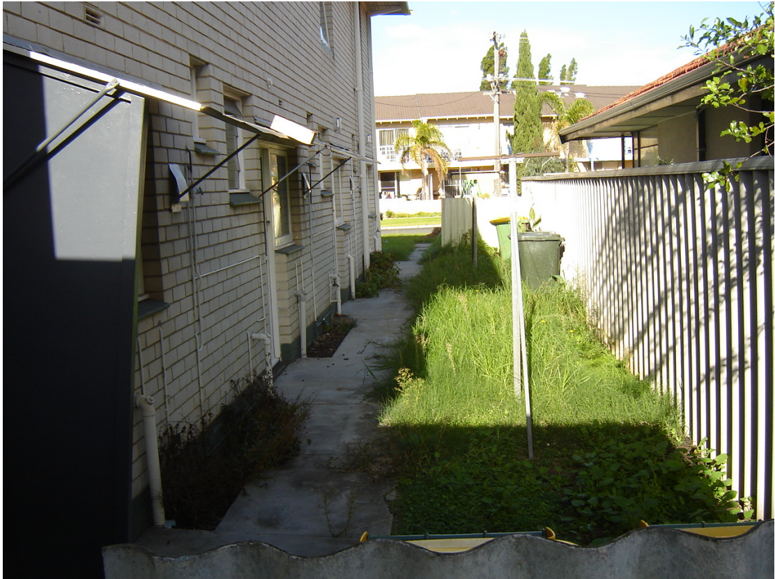
Side of building showing location for proposed bathrooms and courtyards
