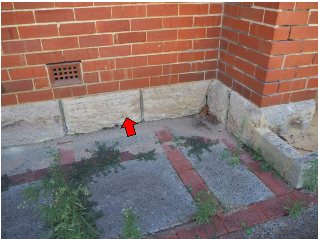
Photo 04 – Example of limestone footing blocks in good condition
