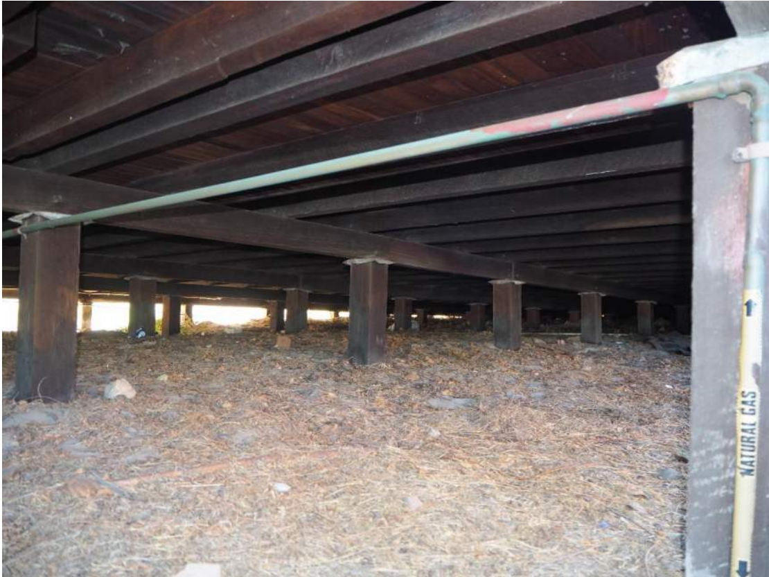
Photo 21 – The floor timbers appeared in good condition.
