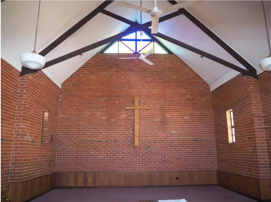
Photo 17 – Church hall walls and ceilings in good condition.
