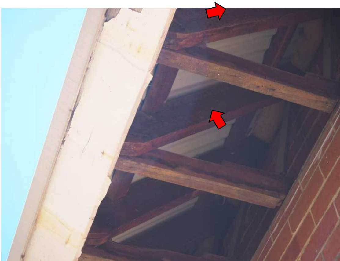
Photo 08 - Roof timber appeared in good condition.
