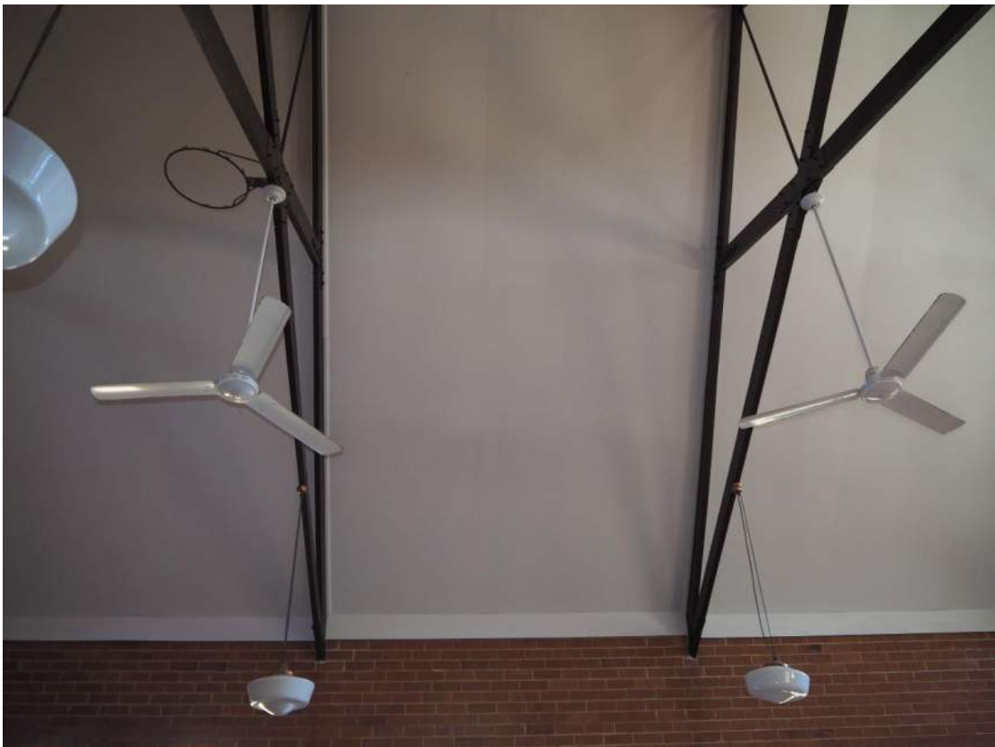
Photo 16 – Church hall ceilings in good condition
