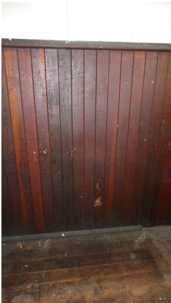
Figure 17: Timber panelling around the Hall
