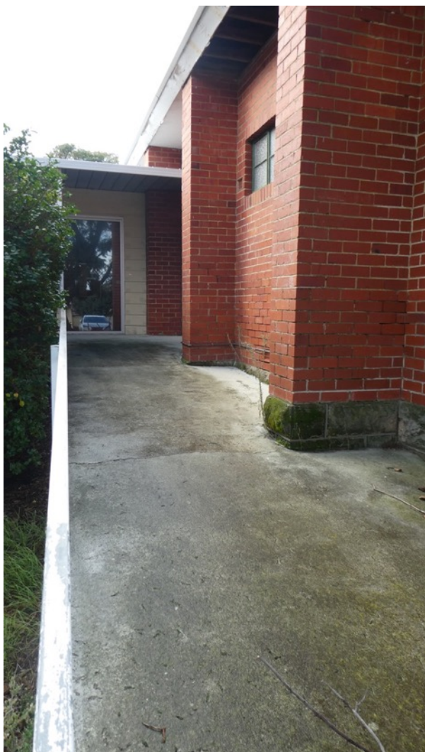
Figure 6: Ramped access into the church addition
