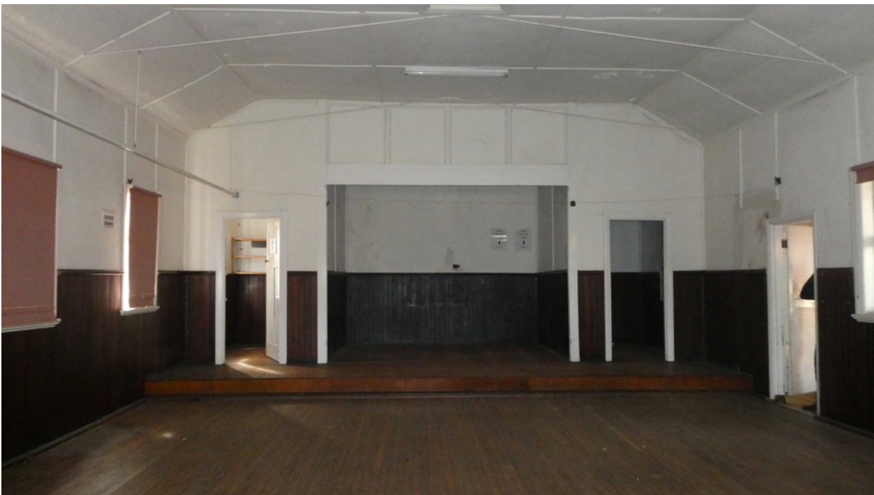
Figure 14: View looking through Durbridge Hall towards the stage
