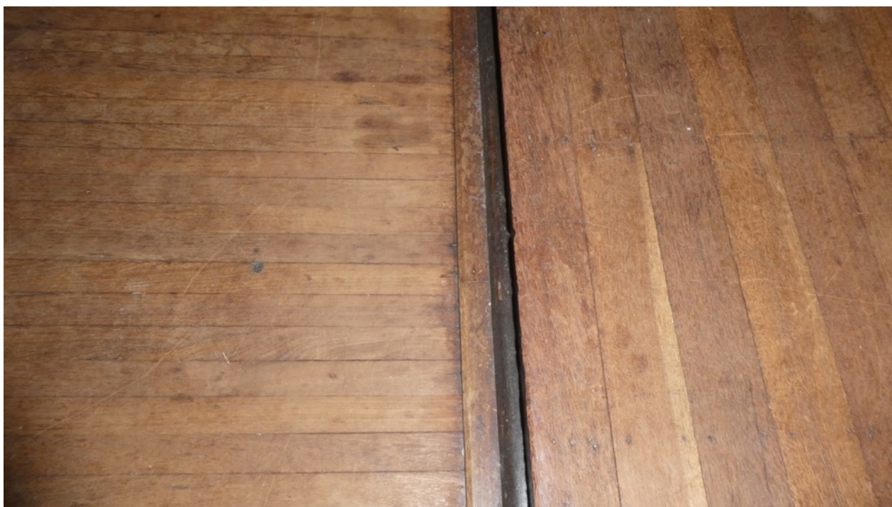
Figure 18: Change in timber floor boards in Hall
