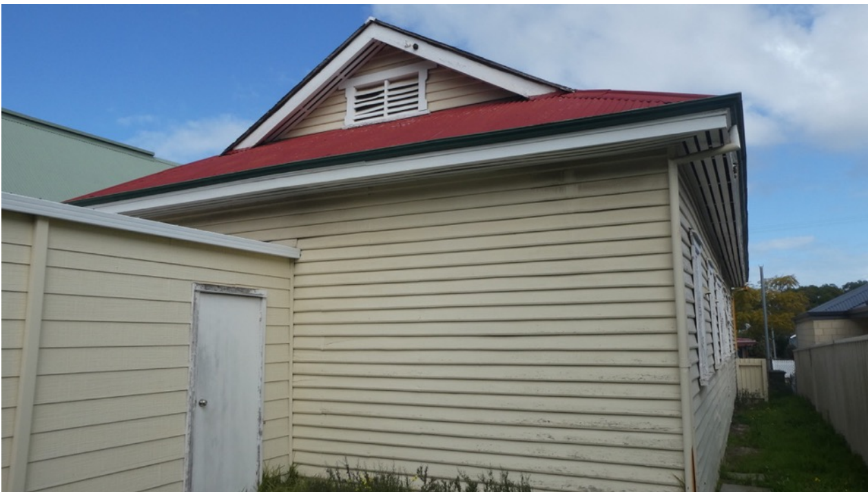
Figure 22: Rear elevation of Durbridge Hall
