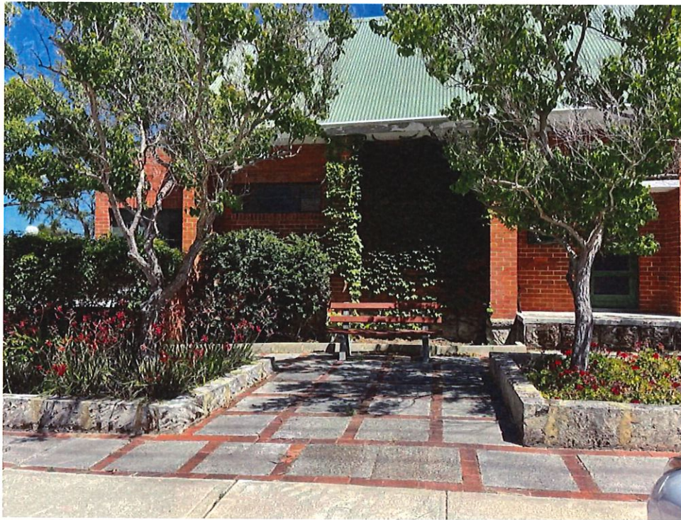
Photograph 3 The eastern façade of the church as viewed from Vista Street. Ivy is growing on the building walls and there are 3 limestone planter boxes along the length of the façade. Griffiths Architects December 2020
