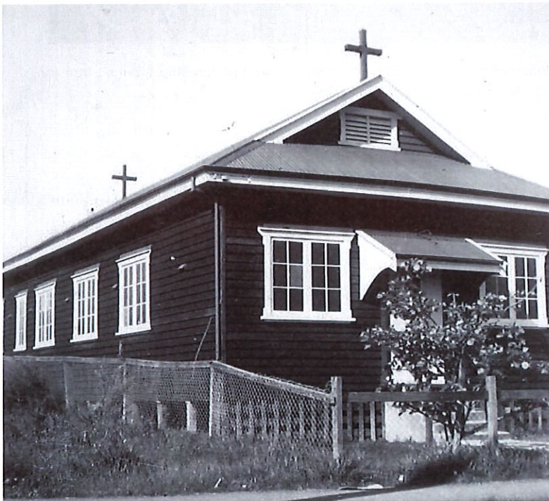
Figure 2 An image of the church taken in 1948, when the weatherboards were oiled and the windows small pane casements. Courtesy Anglican Diocesan Trustees.
