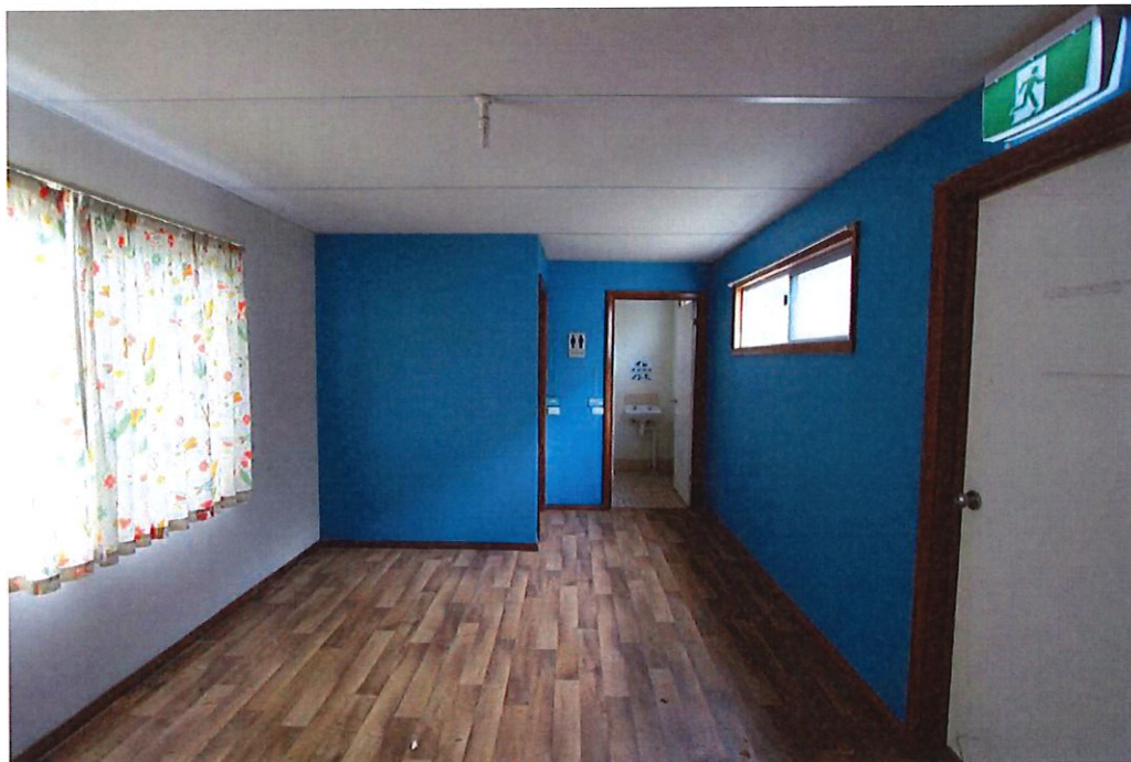
Photograph 10 Toilets at the northern end of the link building. Griffiths Architects May 2021
