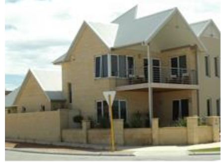
Example of primary and secondary street fencing
