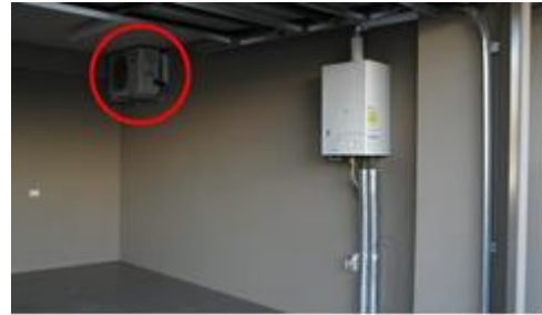
Air conditioning plant located within garage
