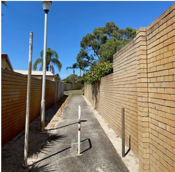
Figure 12 Images of PAWs Showing Insufficient Clearance Around Bollard Structures for Universal Access
