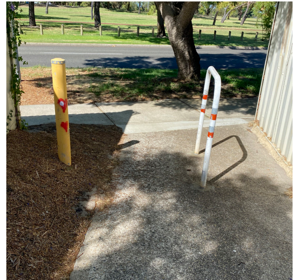
Figure 12 Images of PAWs Showing Insufficient Clearance Around Bollard Structures for Universal Access
