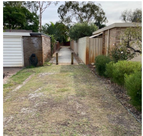
Figure 12 Images of PAWs Showing Insufficient Clearance Around Bollard Structures for Universal Access
